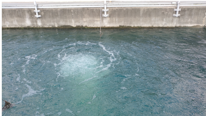
Pictured (above): SET installed a mixer in one of Lawrenceburg's chlorine contact basins; (below): The basin two weeks later
