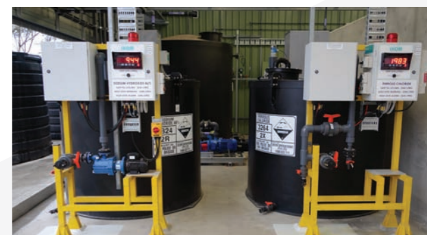
Ixom Bullet™ self-bunded chemical dosing system (no requirement for expensive concrete bund)
