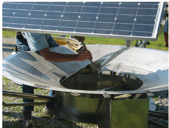
Impeller Removal For Buildup Below Impeller
