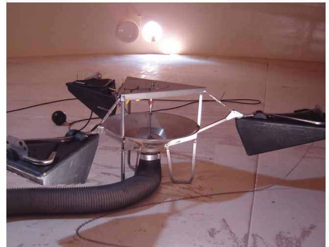
Machine resting on floor ready for water.
