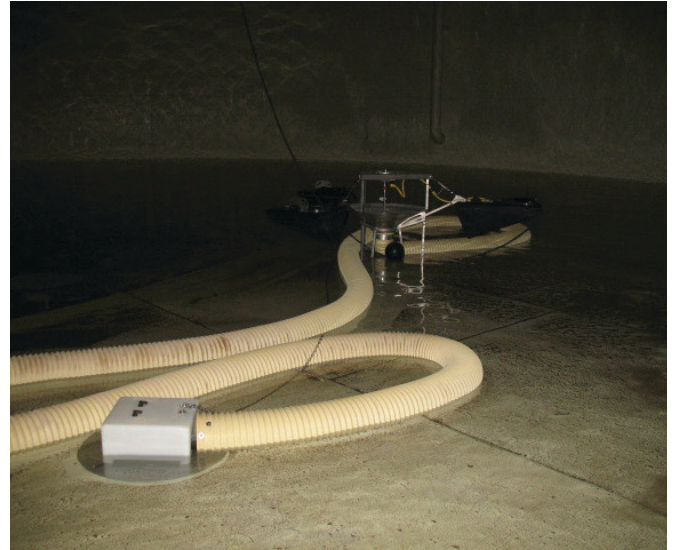
Machine resting in drained tank.
