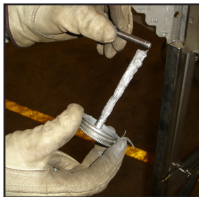
Applying Anti-Seize To The Bolts
