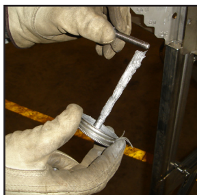
Applying Anti-Seize To The Bolts
