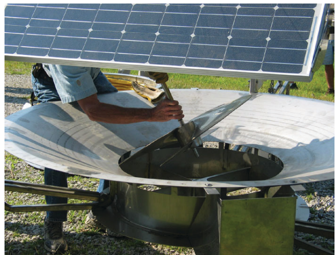
Impeller Removal For Buildup Below Impeller
