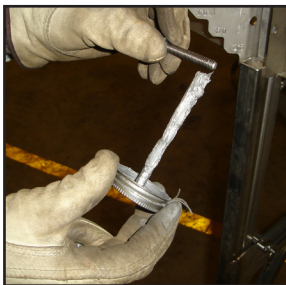
Applying Anti-Seize To The Bolts
