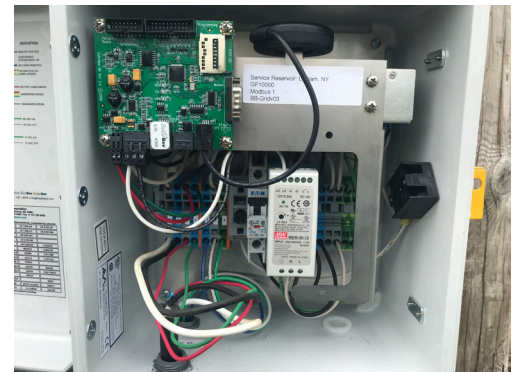
Electronic Control Box of a Service Reservoir
