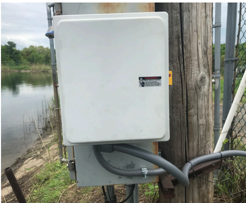
Electronic Control Box of a Service Reservoir
