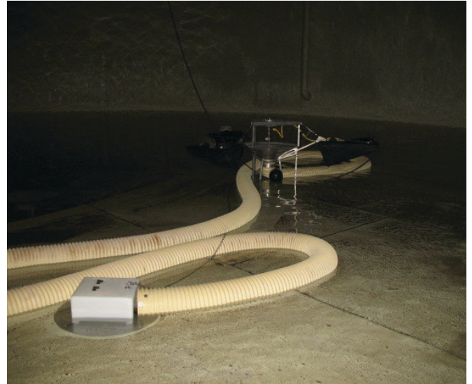
Machine resting in drained tank.
