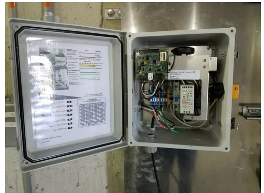
Electronic Control Box in Tank Reservoir
