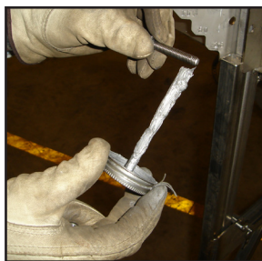
Applying Anti-Seize To The Bolts
