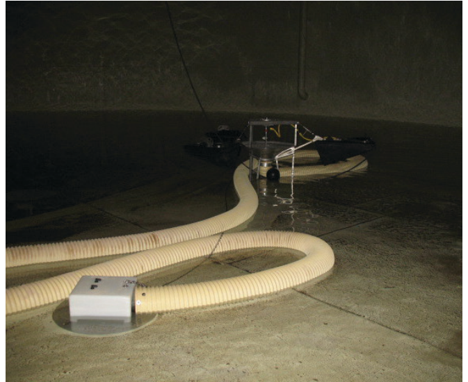
Machine resting in drained tank.
