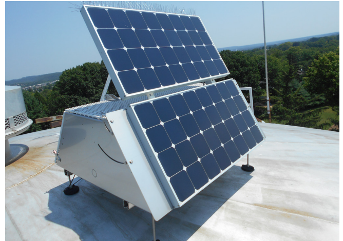
Battery Electronic Controller
