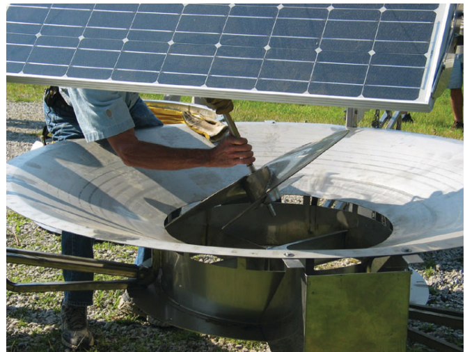
Impeller Removal For Buildup Below Impeller
