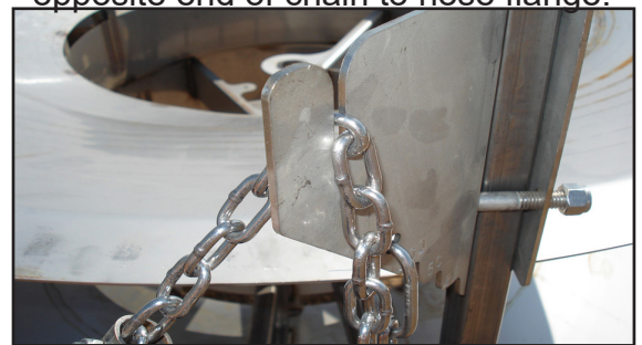
Marker chain slipped into chain bracket slot.
