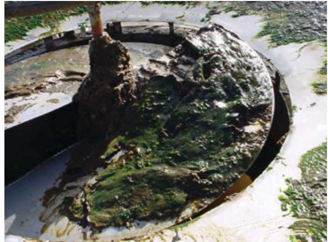
Machine With Buildup On Impeller
