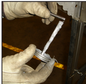
Applying Anti-Seize To The Bolts
