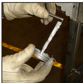
Applying Anti-Seize To The Bolts
