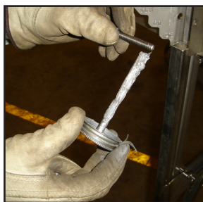
Applying Anti-Seize To The Bolts
