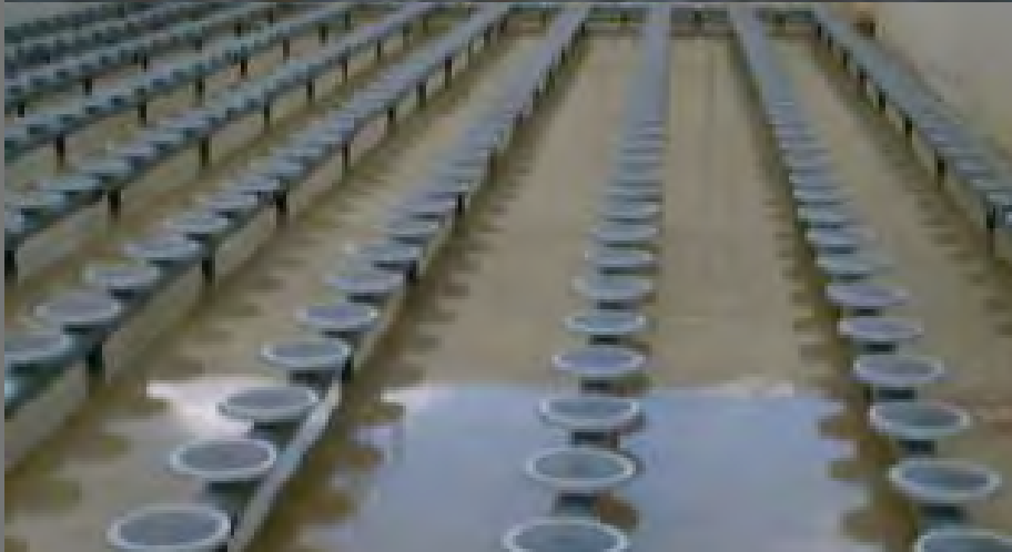
Diffused Air Aeration (fine bubble / coarse bubble)
