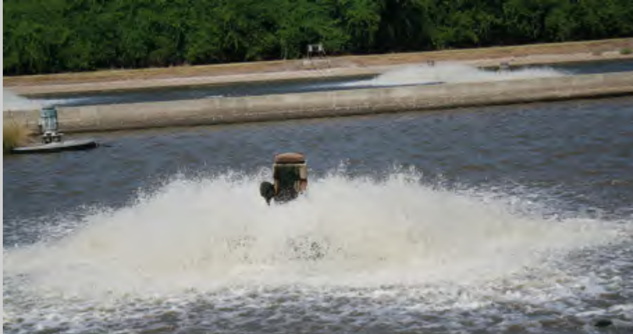
Splasher Type Aerators
