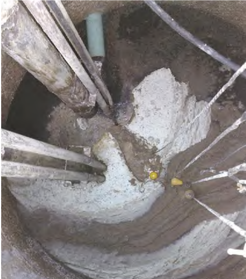
Before startup of AP500 in Wet Well
