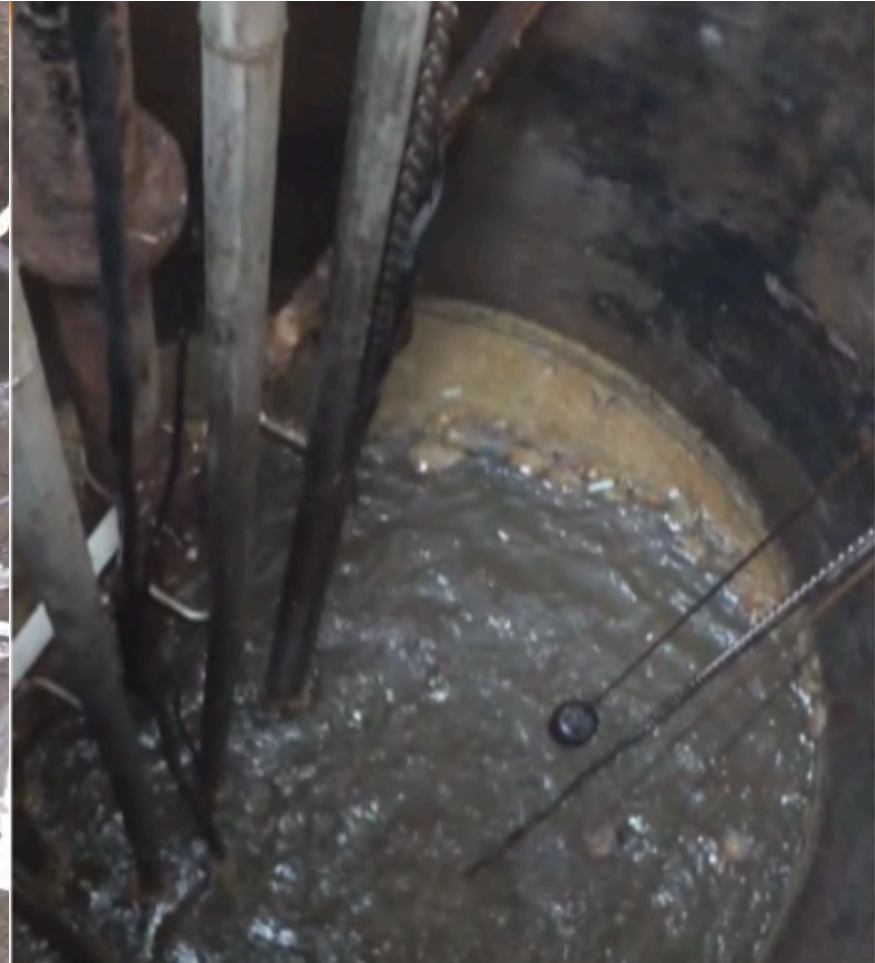
After startup of AP500 in Wet Well
