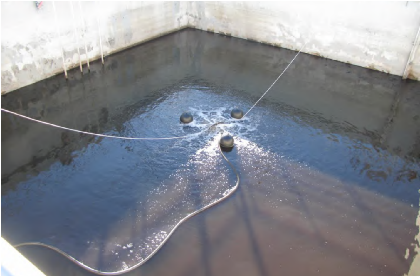
AP7000F Floating Style Mixer in basin, after 2 days
